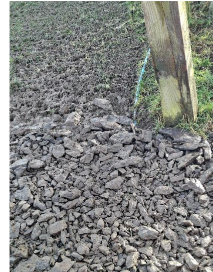
Image 30: Part of the water pipe hidden by Made Ground paved with coarse gravels.
