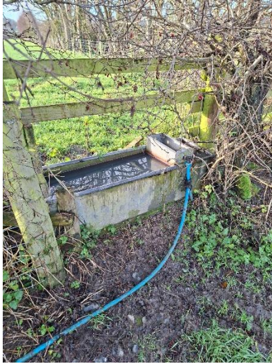
Image 31: Water pipe connected to a trough located on the northern corner of Area C.
